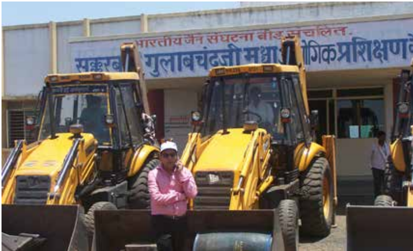
Poclains and JCBs mobilized for the ground water restoration and desilting project in Beed.
