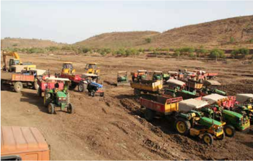
Poclains and JCBs at work for depositing 20 lakh cubic metres of silt.
