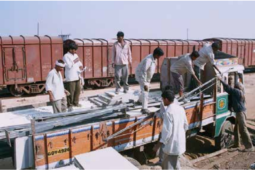
The material was coded, dismantled, and transported from Gandhidham, Gujarat to Jammu in three trains.
